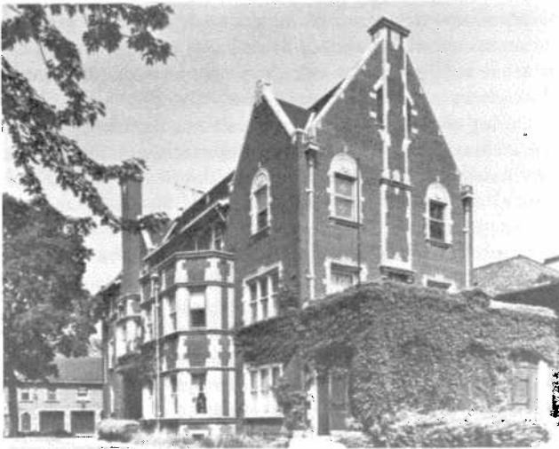
The suburban character of Kenwood derives from the many large houses set on spacious lots, such as the house at 4940 Greenwood Avenue which was designed in the Tudor style. (Barbara Crane, photographer)
